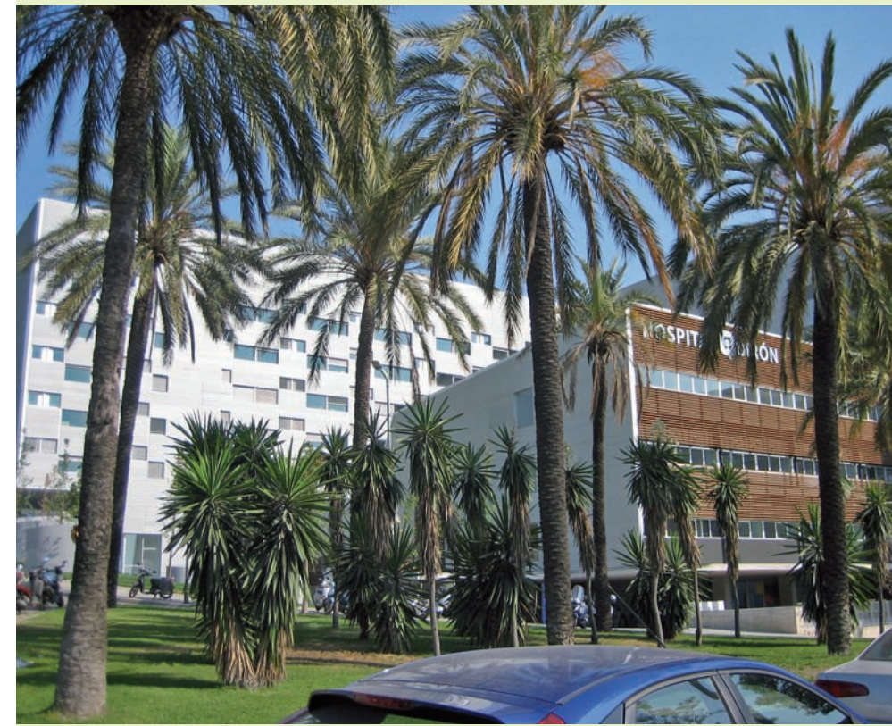
Hospital Quirón Barcelona
